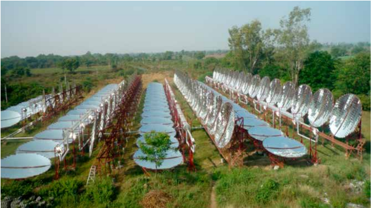
Parabolic solar collectors power the air conditioning system at Muni Seva Ashram Hospital in Goraj, India. (Photo: Urvish Dave's Blog & Muni Seva Ashram – Goraj)
